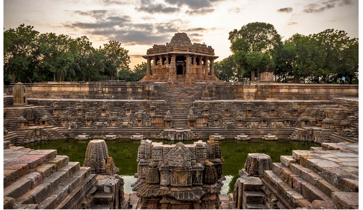
Construction of a stepwell (vav) for the community
